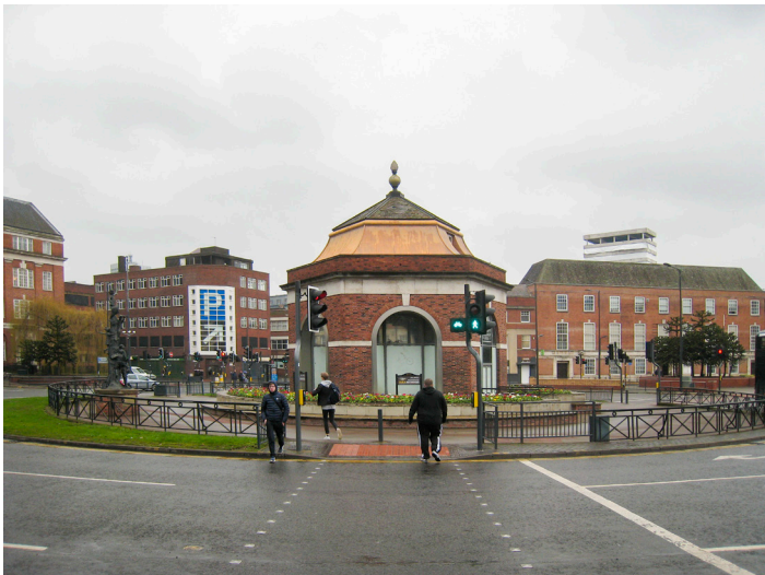
Eastgate and St Peters St: excessively wide for traffic
