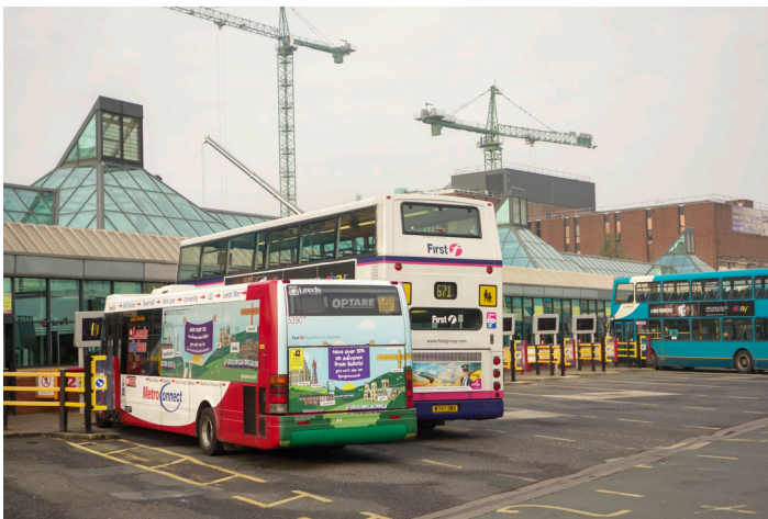
The Bus Station: needs reconfiguring
