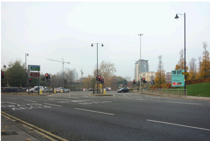
East Street: an over-engineered highway
